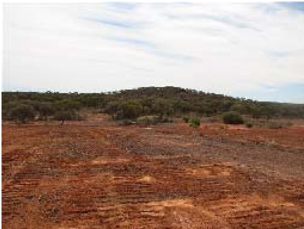
Hepi project - 2.5 Hectare clearing for trial pit
